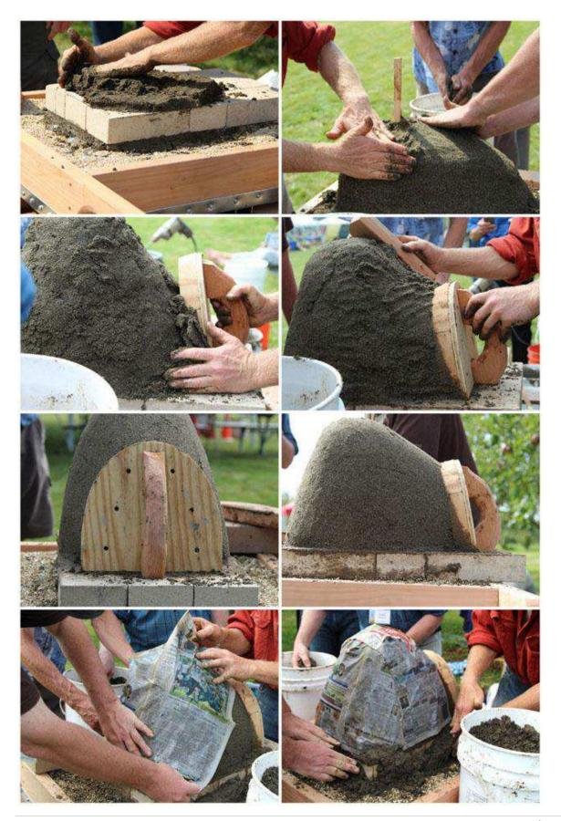
To create the interior dome, we will mix some water with sand, just like building a sand castle. You can cheat a little by adding a small amount of clay soil so the form holds up easier, but is still loose enough to be scooped out later.
