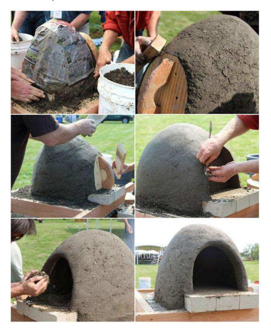
The purpose of the thermal layer is to hold heat in its dense mass. Use the clay-sand mix we made earlier, take one handful at a time, and press it down to form a 2"-3" shell outside the sand form. Be careful not to press into the sand form, which would cause the form to shift.
